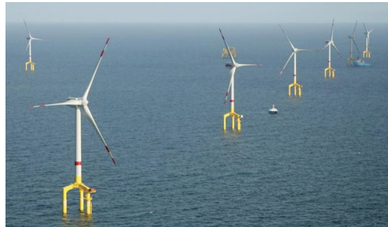
Figure 2. Wind turbines (typ BARD 5.0) in the German North Sea, wind park BARD Offshore 1 [www.bard-offshore.de].
