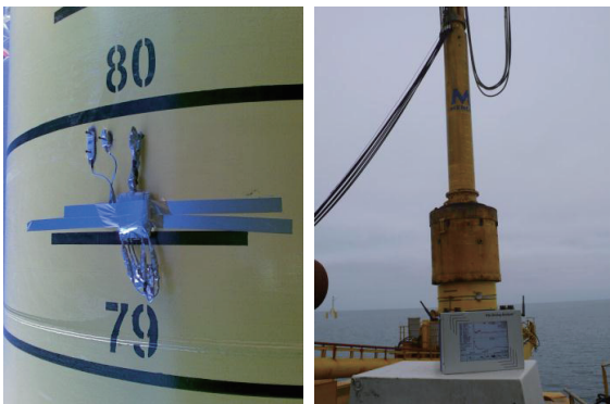
Figure 4. Measurement equipment attached to the pile after bolting (left) and during driving (right).
